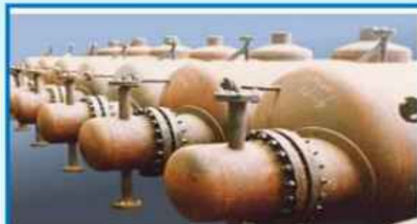
熱油蒸氣器(Hot Oil Evaporator)
